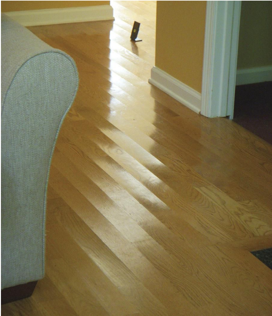
Moisture-related issues can lead to installation failures such as the cupping seen in this hardwood floor. Photo courtesy of National Wood Flooring Association.
