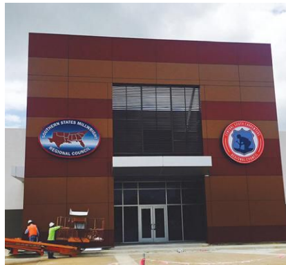
The Carpenters and Millwrights Training Center has moved to a new 52,000 sq. ft. facility in Pasadena, Texas.
