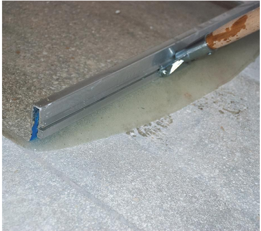
Applying an epoxy moisture barrier over concrete. Photo courtesy of MAPEI.
