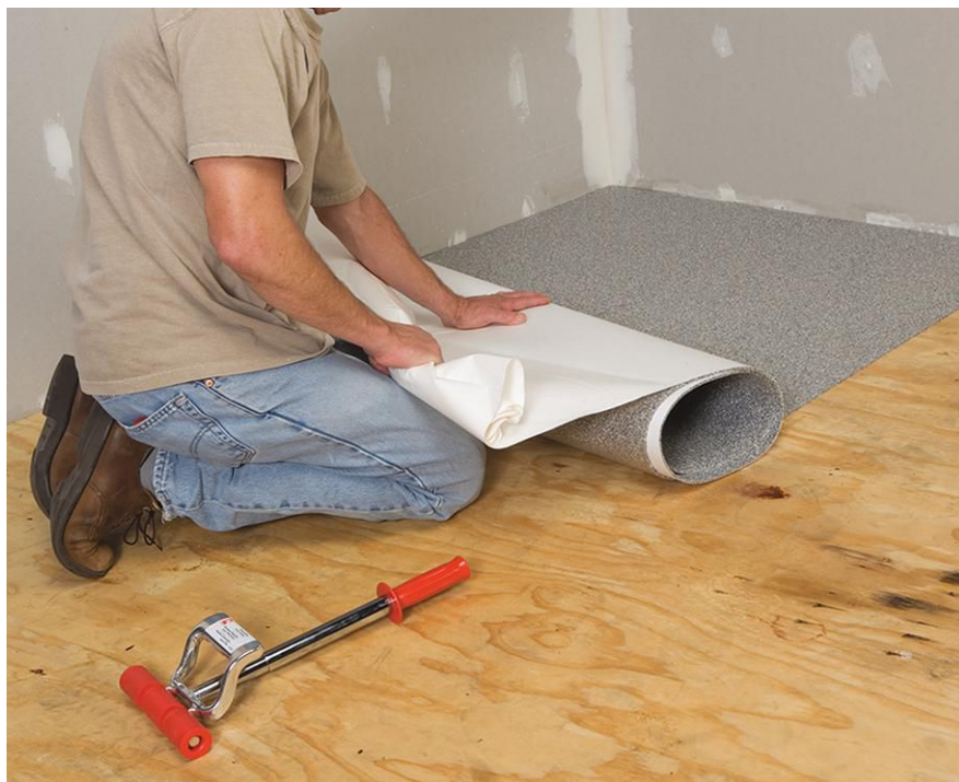
Custom Building Products' sound control offerings include Crack Buster Pro Crack Prevention Mat Underlayment and EasyMat Tile & Stone Underlayment. Photo courtesy of Custom Building Products.
