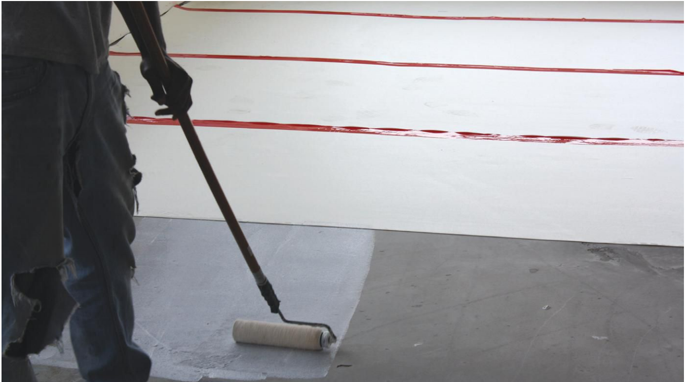
Along with its wide range of flooring adhesives, DriTac now offers two underlayments: DriTac 8301 Impact for resilient floor installations and DriTac 8302 Double Impact for wood and laminate floor installations. Photo courtesy of DriTac.
