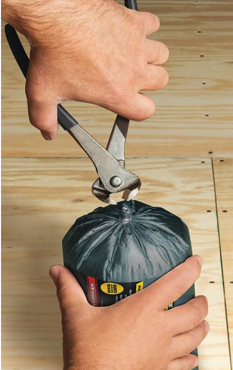
First snip the tail on the pouch, then squeeze out the adhesive.
