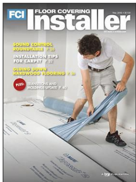
On the cover: Applying MAPEI's Mapesonic 2, a lightweight, load-bearing peel-and-stick sound reduction and crack isolation membrane. Photo courtesy of MAPEI.
